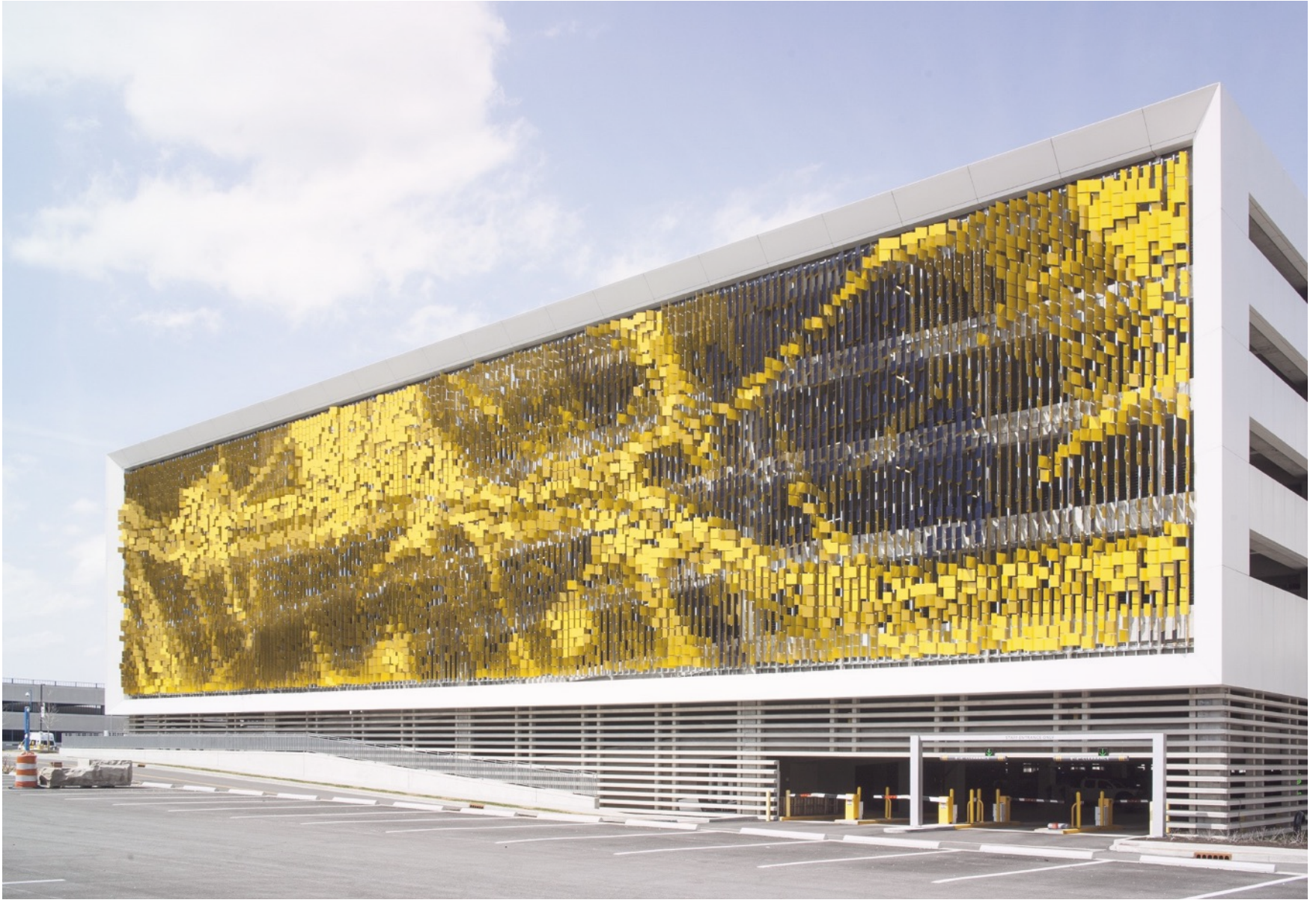
Urbana: Sidney & Lois Eskenazi Hospital, Parking Structure Art Facade, Indianapolis, USA // f.: archdai.ly
