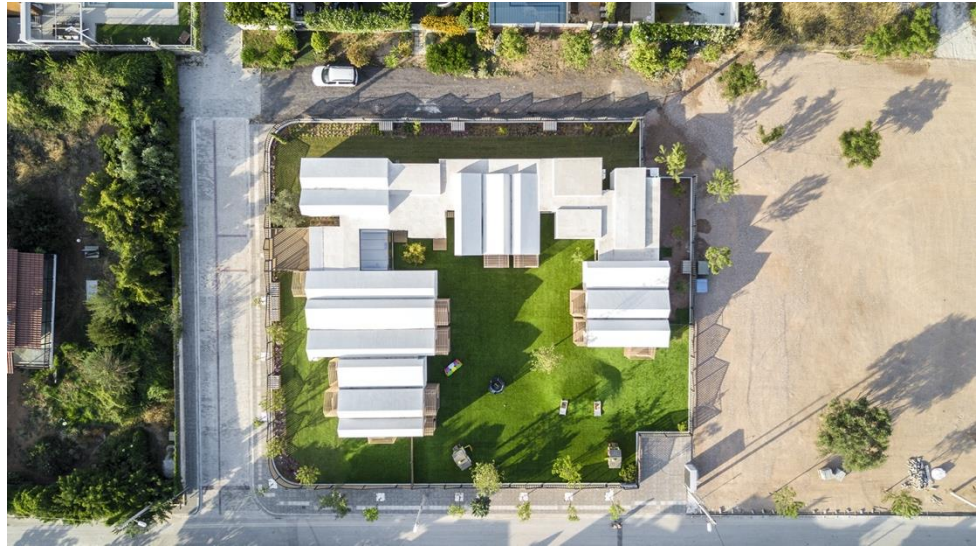
▪ Glyfada Óvoda. https://www.detail-online.com/blog-article/municipal-kindergarten-in-glyfada-by-klab-architecture-31236/ (Utolsó elérés: 2021. 03. 28.)
