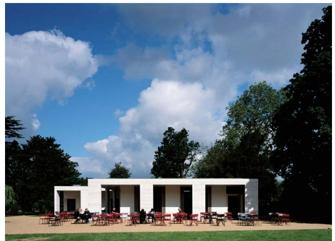
Chiswick House Cafe, Caruso St. John, 2010
