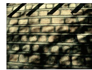
The students needed to peel and cut the trunks in 50 cm long pieces. The clay was made in situ with the use of sand, fjord water and marine clay, though originally in this technique clay with water from the glacier time, taken from the soil, was used. The majority of the stones used were selected and carried from the fjord shore next to the building site, only the especially big and flat pieces came from a bit further, from a local quarry.
