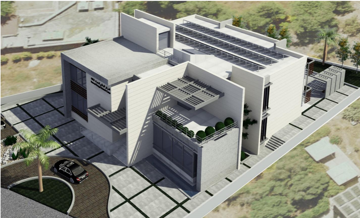
Figure 4: Building visualization (Source: Imad Al-Dabbas Office (2016))
