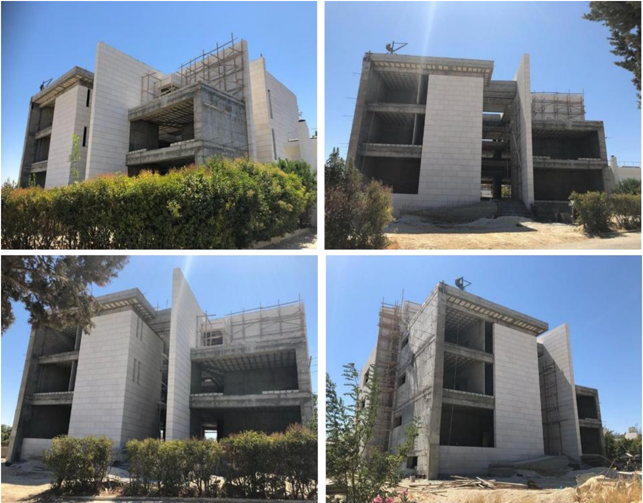
Figure 11: Construction phase (Source: Imad Al-Dabbas Office (2021))
