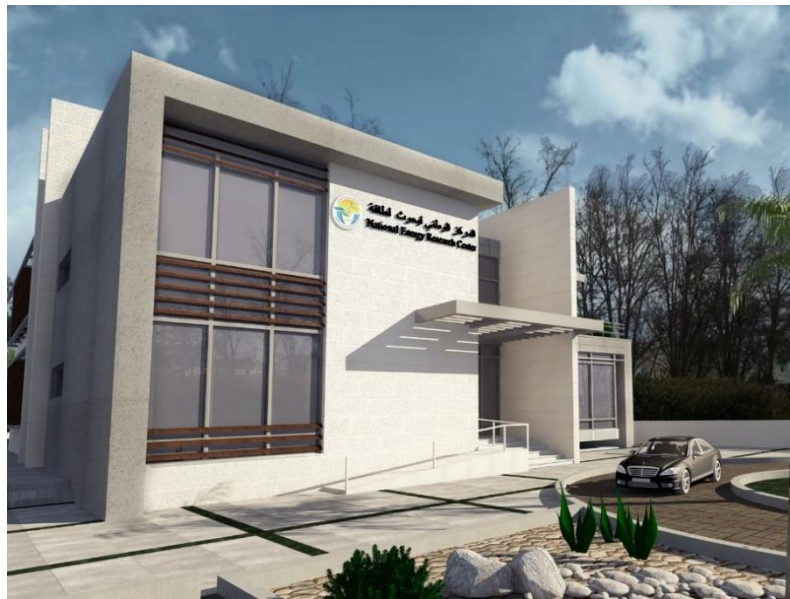
Figure 1: Building visualization (Source: Imad Al-Dabbas Office (2016))
