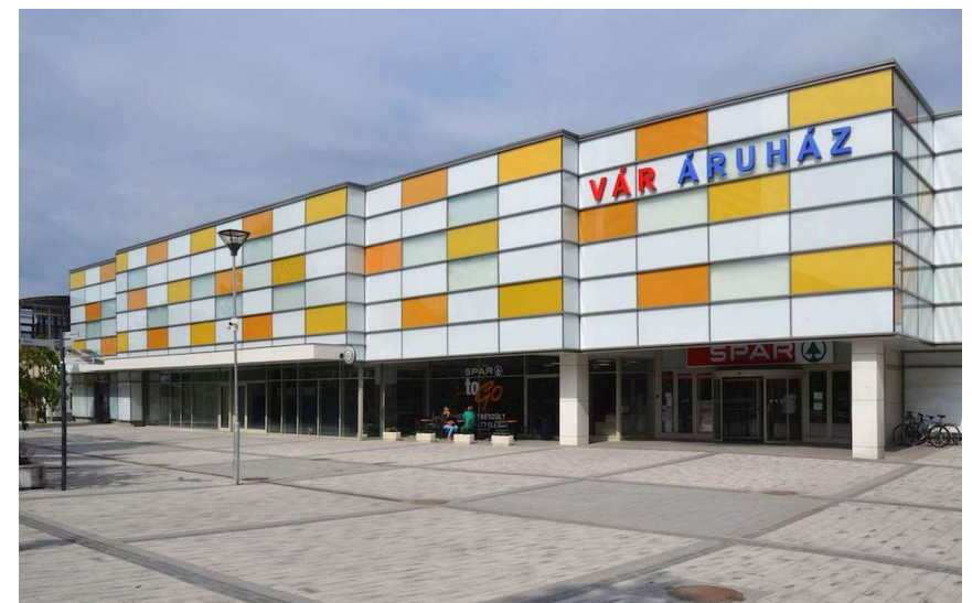
Vár Áruház department store after the reconstruction
