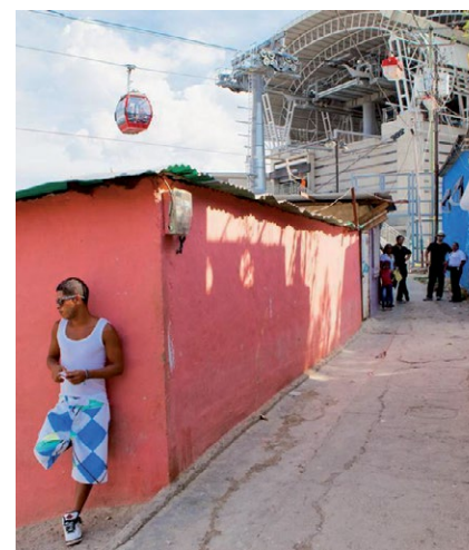
Kábeles Metro / San Agustín, Caracas, Venezuela / Alfredo Brillembourg and Hubert, Urban-Think Tank (U-TT), Klumpner, 2007–2010 —moma.org
