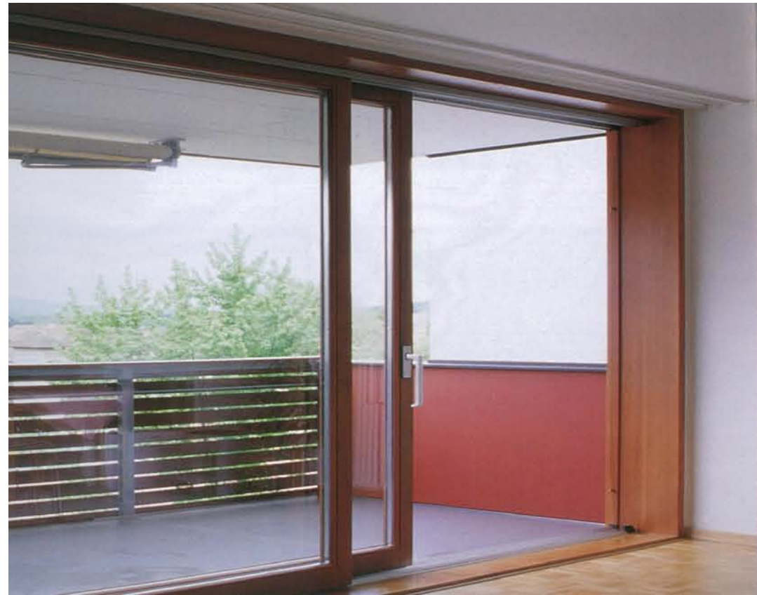
Facade renovation of Dettenbühl Development, 1996
