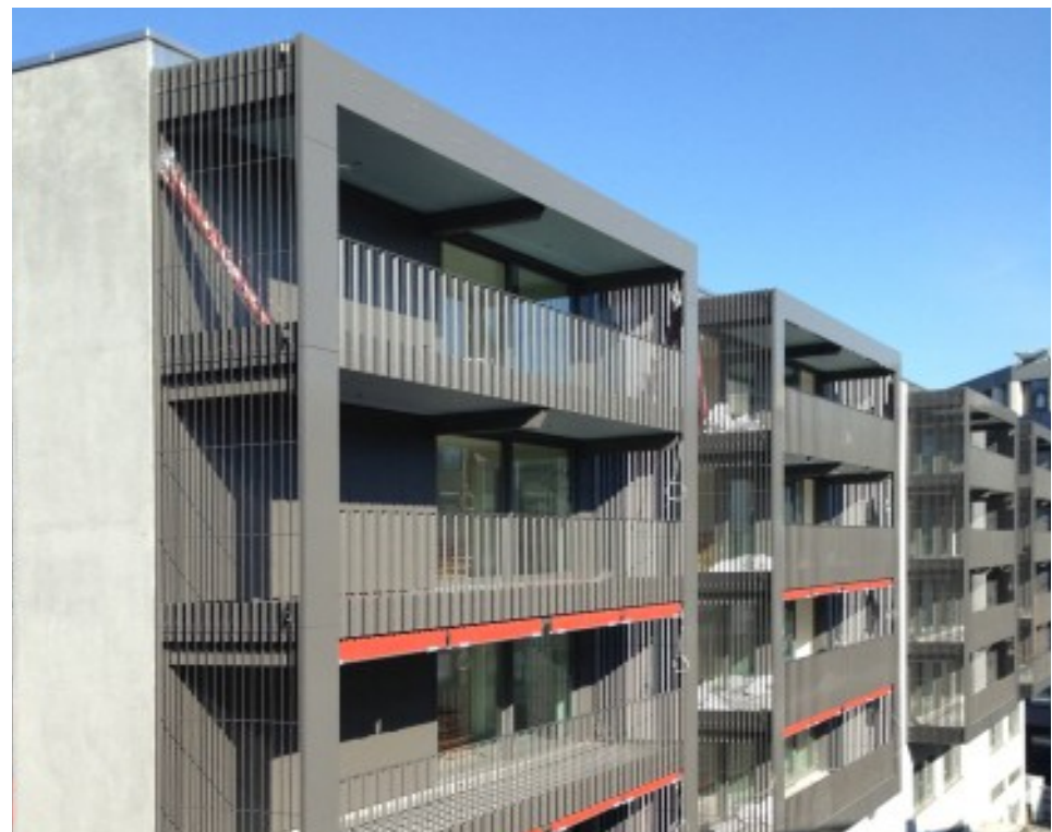
Conversion of a storage building, Giesshübel, 2013
