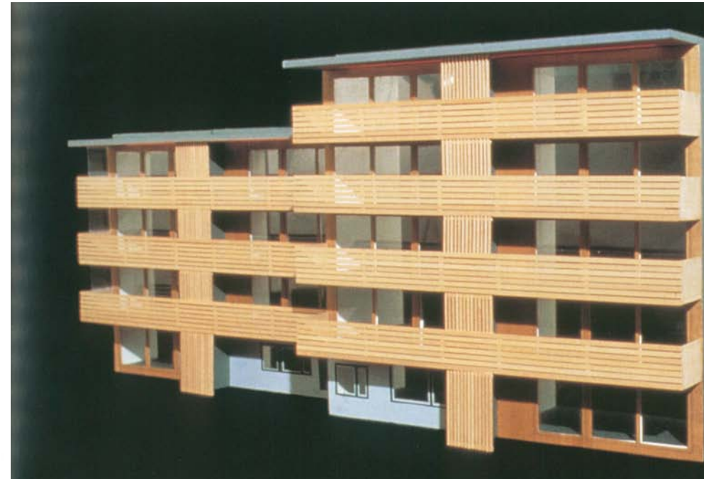
Facade renovation of Dettenbühl Development, 1996
