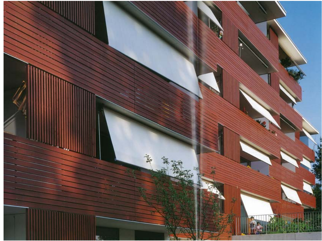
Facade renovation of Dettenbühl Development, 1996
