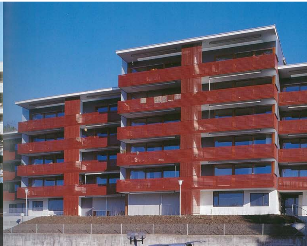
Facade renovation of Dettenbühl Development, 1996
