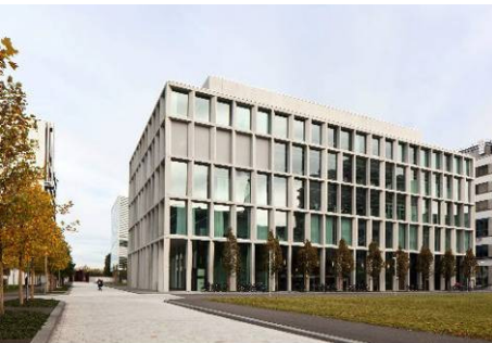
Chipperfield: Laboratory building, Basel, 2010
